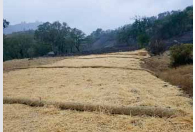
Loose straw mulch and straw wattles are among the methods used to prevent soil erosion and debris runoff at Kimball Reservoir following the Tubbs Fire. Photo from Calistoga Public Works Staff
