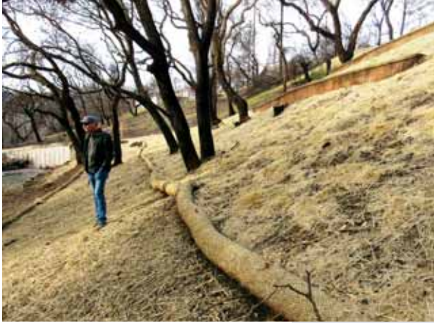
Loose, straw mulch with straw wattles placed along the slope contour. Photo by Julie Evens
